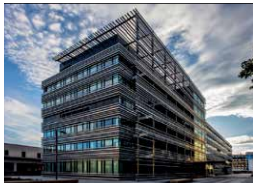
Neues Technologiezentrum am Headquarter
